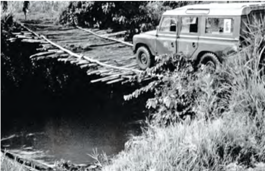
Photo Credit: In Ethiopia, there were limited roads which were sometimes impassable. But the bridge shown here was crossed four times in 1974, Ethiopia, 1974. World Health Organization. http://www.who.int/features/2010/smallpox/work_conditions/en/index1.html
